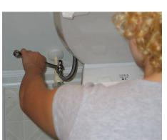
3. Install the "Tee" supplied with the USABidet® and reinstall the fitting on the flexible line to the toilet on the upper connection of the "Tee."
